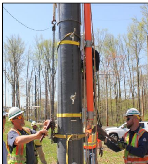
Figure 24: Compressing the joint from the ground using 2-ton lever hoists.
