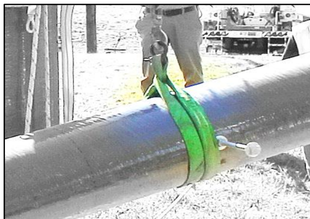
Figure 19: A short lifting sling installed below a step bolt will prevent slippage.
