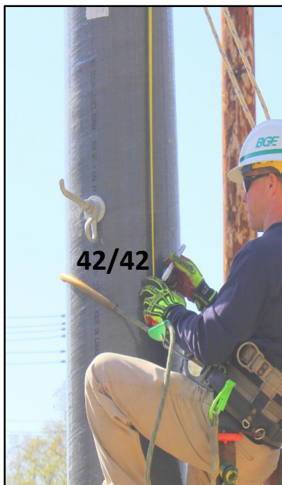
Figure 11: Measuring and marking the clamp assembly locations along the gin pole.
