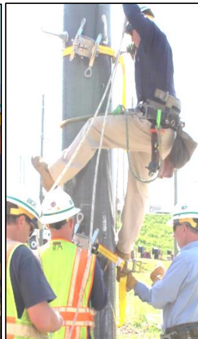
Figure 12: Installing a clamp assembly in preparation for mounting the gin pole.
