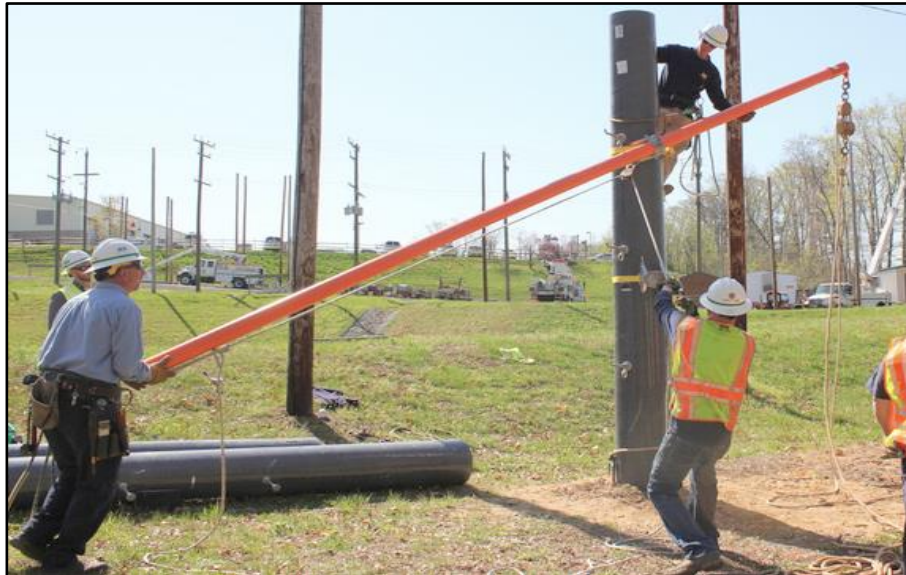
Figure 14: 3-sheave blocks and a tag line are attached to the gin head before raising the gin into the vertical position.
