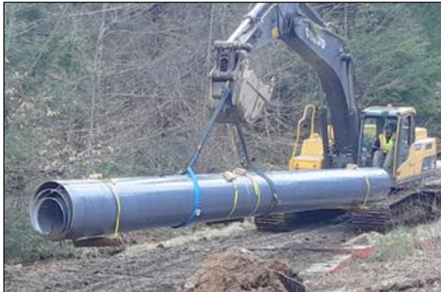
Figure 17: Nested 90 ft. [27m] pole crawling into remote installation site.
