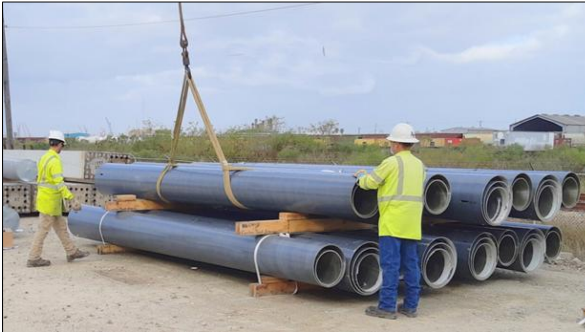
Figure 14: Storing RS poles with wood dunnage between layers and well spaced rows for efficient categorizing and loading.
