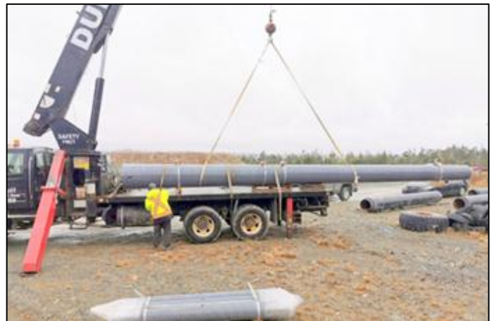
Figure 9: Unloading a pole set using two slings and two points of contact.
