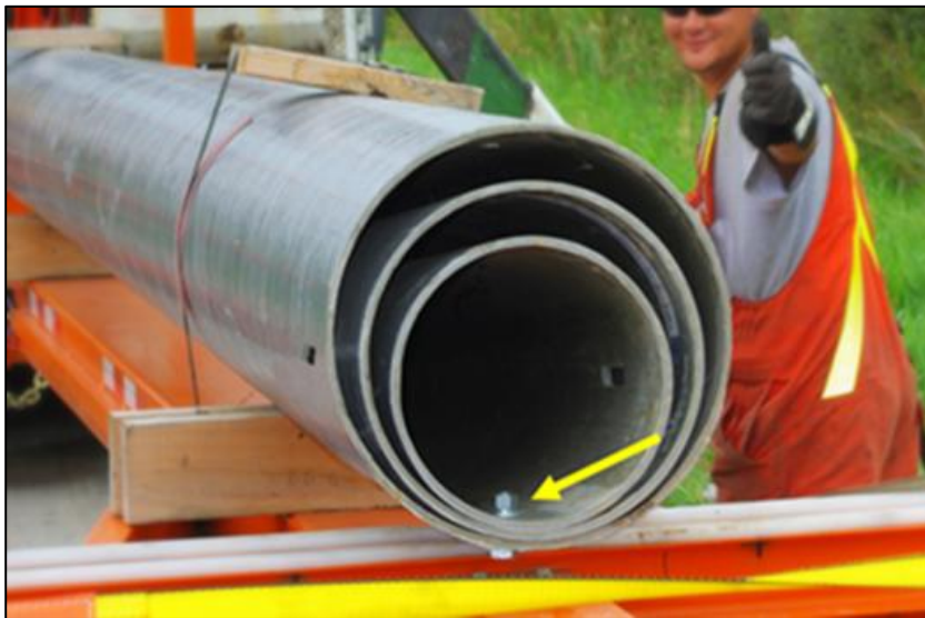
Figure 5: Shipping Bolt securing the nested modules during transportation.
