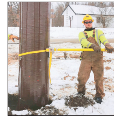
Figure 27: RS Poles Can Be Turned Easily Using a Pole Cant
