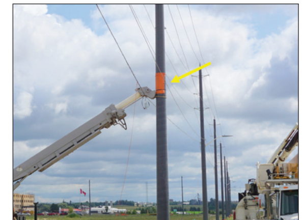
Figure 23: Temporary Rubber Matting to Protect the Pole Surface From the Boom
