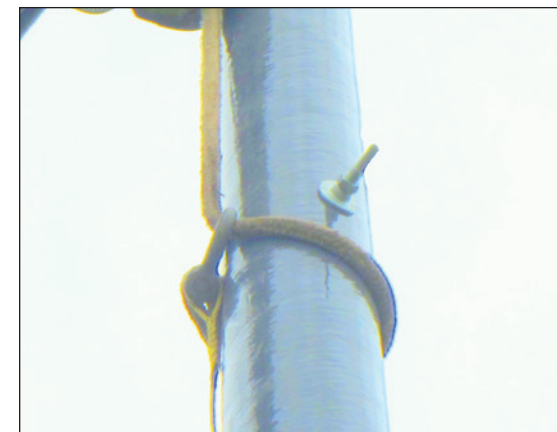
Figure 22: Temporary Through Bolt to Prevent Sling Slippage
