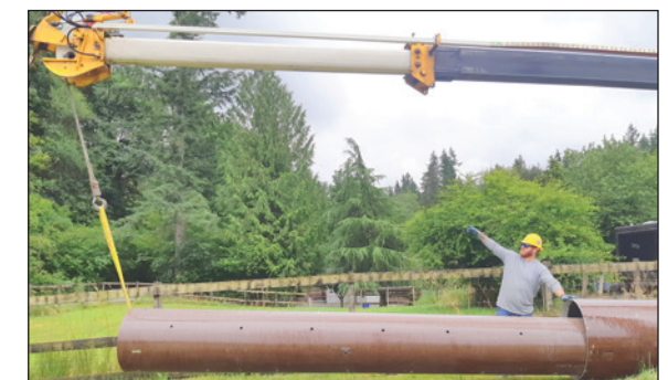
Figures 3a and 3b: A Derrick Boom Truck Lifting Up and Outwards to Unnest Modules and Prevent Scratches
