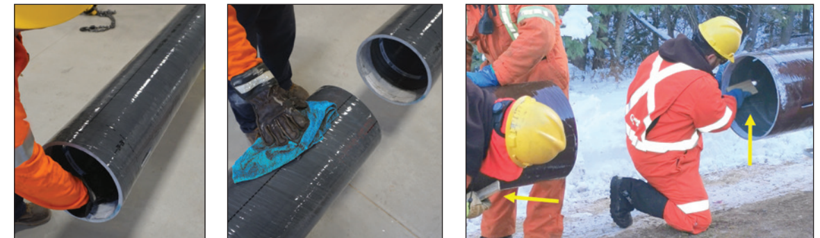
Figures 7a, 7b and 7c: Wiping the Inside Surface of the Upper Module and the Outside Surface of the Lower Module
