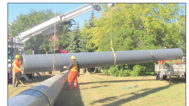
Figures 4a and 4b: Small Modules Being Unnested and Laid Out for Assembly
