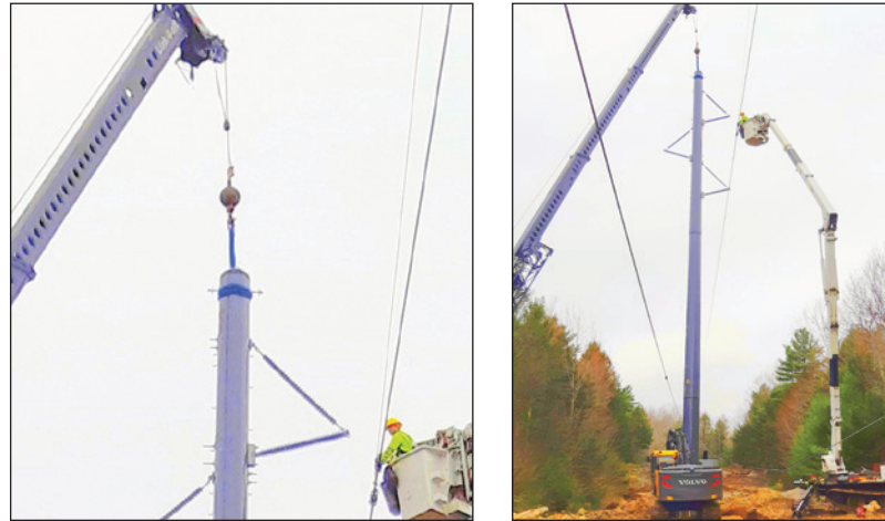
Figures 24a and 24b: Crane With a Choker Sling Installing a 95 ft. [29m] Pole for a 115kV Circuit
