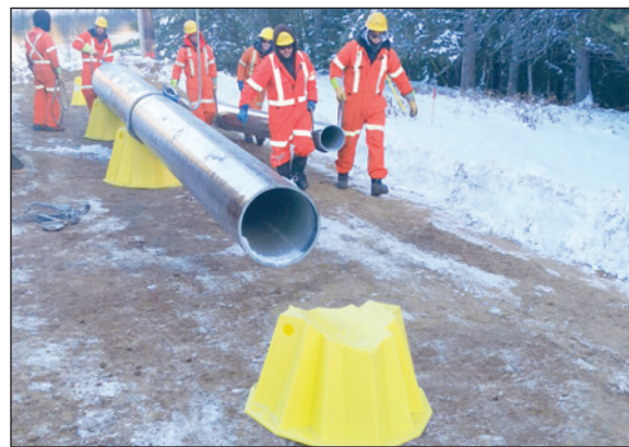
Figure 5b: An RS Pole on Pole Stands
