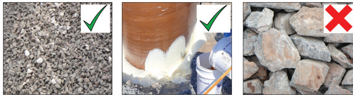
Figures 29a, 29b, and 29c: Examples of Acceptable and Unacceptable Backfill Options
