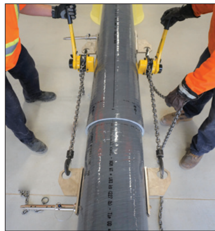
Figure 12: Equal Assembly Force Being Applied to Both Sides
