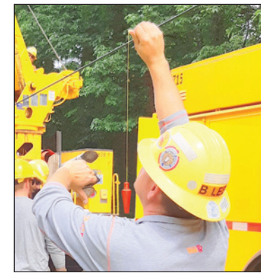
Figure 26: Using a Plumb Bob to Vertically Align a Pole
