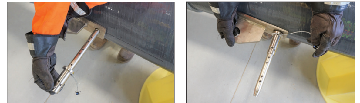
Figures 10a and 10b: Installing the Retention Collar and Determining the Correct Set of Holes for a Tight Fit
