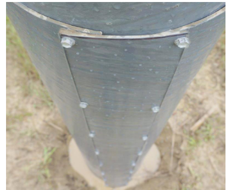
Figure 13: Securing the cover strip.
