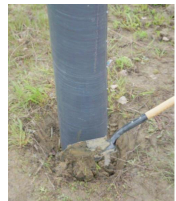
Figure 9: Trenching around the base of the destination pole.
