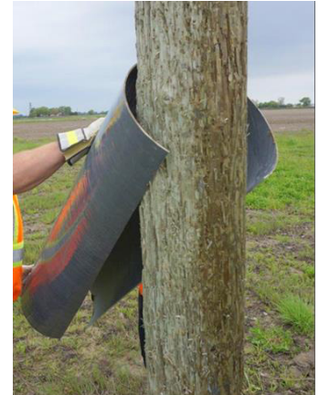
Figure 10: Spreading the primary shield while pushing inward and upward onto the destination pole.
