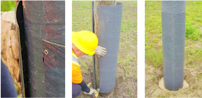
Figure 12: Secure the primary shield with flat head construction screws.
